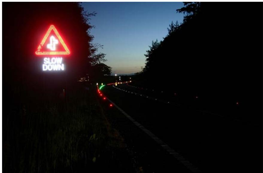
at either side of the road just before the connecting roads joined the main A41 carriageway. The studs were programmed to constantly emit low level light during the hours of darkness and if a vehicle were to exceed the speed limit on passing either of the VAS signs they would flash “Slow Down” with the hardwired studs automatically changing to full brightness, dramatically increasing the driver’s visibility of the road ahead.
