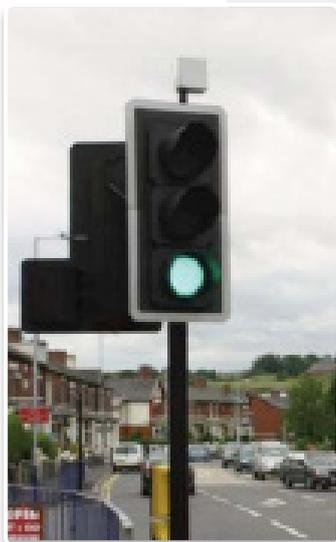
The in road sensor communicates wirelessly using a low power, highly secure and unique radio protocol, to send time stamped detection data to the M110 Access Point, within a range of 30 to 40m away, that forms the heart and hub of the system. The Access Points are usually mounted on top of a suitably positioned signal head.
