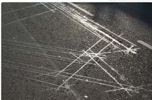
newly installed loops and so the cycle continues. Other locations where the inductive loop creates an issue are those where detection is required in alternative road surfaces such as block paviers or where existing iron work in the road prevents the loop being installed in the correct location.
