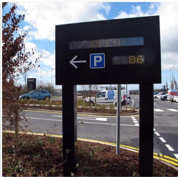
Parking guidance systems such as capacity counting systems in conjunction with Variable Messaging Signs (VMS) and bay monitoring can help in this regard and make your parking more flexible and open up other possibilities to maximise the space available.
